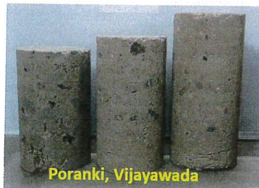
Photo. 20 Condition of stabilised cores after durability test (Samples collected in the year October 2020)
